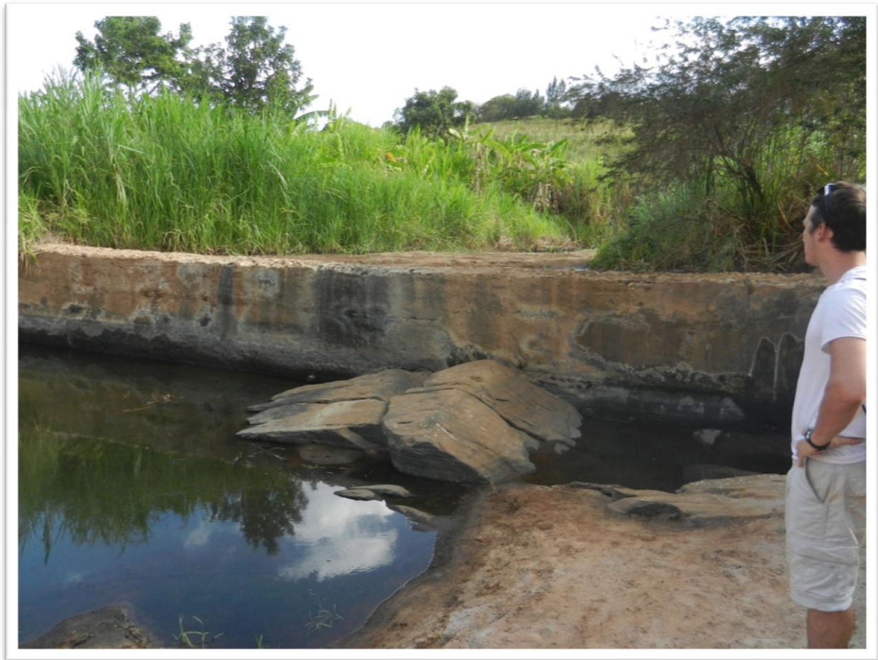
Figure 1: Nzaaya Muisyo Dam #67 located at 01 41.215 S latitude and 37 24.581 E longitude. The dam is 2 meters high above bedrock, has a 21 meter wide spillway, backs up sand for 230 meters, holding approximately 5000 cubic meters of sand and 1750 cubic meters of water in the pore space at full capacity. Note that behind the dam are abundant, flourishing stands of Napier grass used for cattle fodder and bananas, which would not thrive in the area without the sand dam. The picture was taken in July 2013 about 2 months after the last of the long rains in May.
