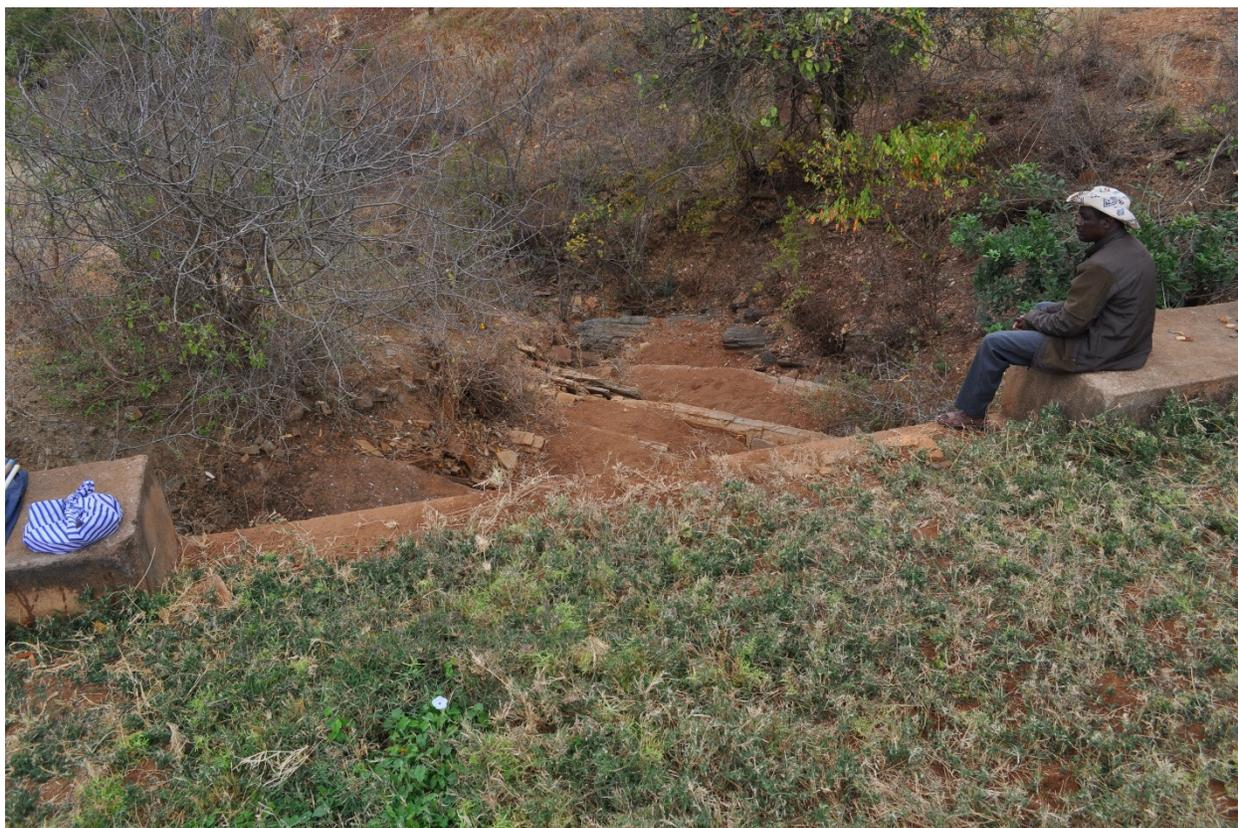
**Figure 4.2: Silted sand dam.** *Some non-functioning sand dams filled predominately with silt, as indicated by vegetation growing upstream of the structures.*
