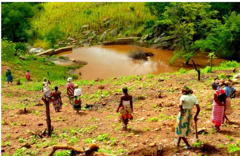
**Figure 2.5: Suspended fines in open pool.** *At the end of a rainy season, some suspended sediment is often left in the open pool upstream of a partially-filled sand dam, and settles out during the dry season.*
