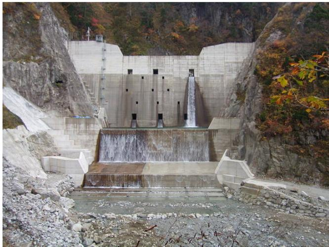
**Figure 6.3: Sabo dam.** *Sand dams might employ drainage outlets like those of this sabo dam, constructed near Toyama, Japan (Shitaka.net)*
