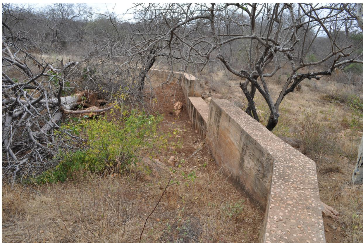
**Figure 6.2: Failed sand dam.** *Sand dams built on rivers without sandy riverbeds will not likely benefit from staged construction.*
