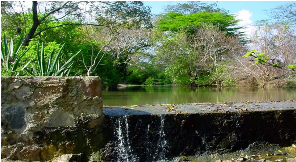
Photo 2: A sand dam in the wet season
