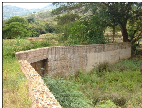
Sand dam in Machakos region
