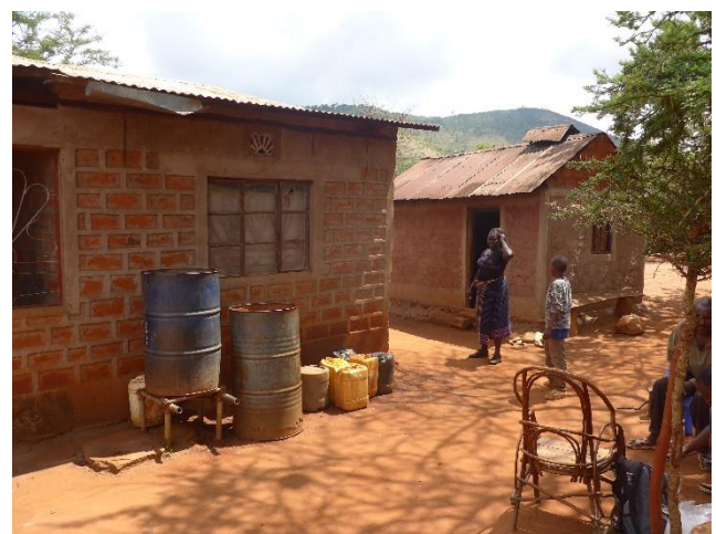
Fig. 5 Rainwater collection system typical of that used during rainy season.
