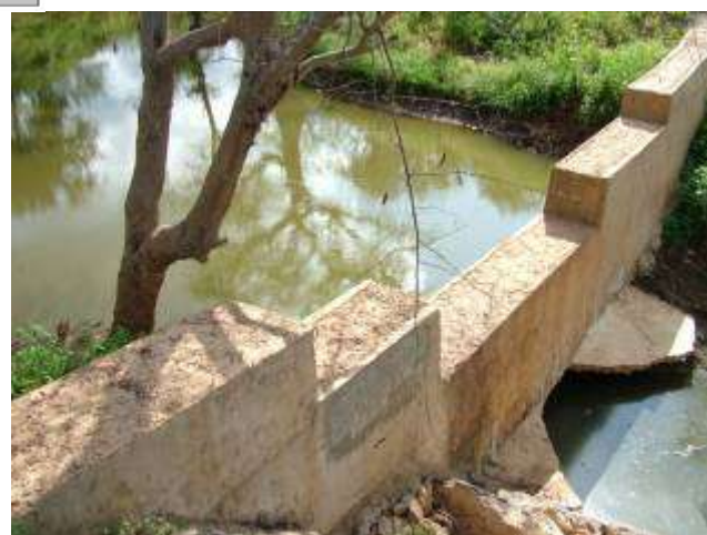
Sections of the apron have been undermined due to foundation and size of the apron being inadequate.
