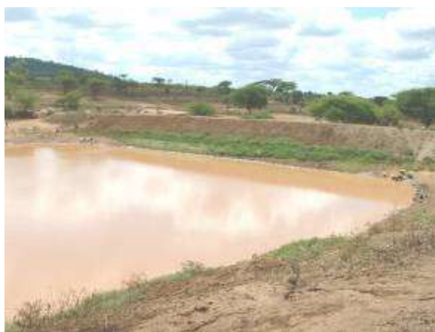
Earth Dam, Kenya. Credit: UDO / EDK
