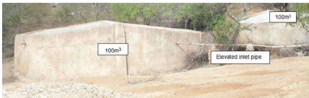
Rock catchment and storage tanks
