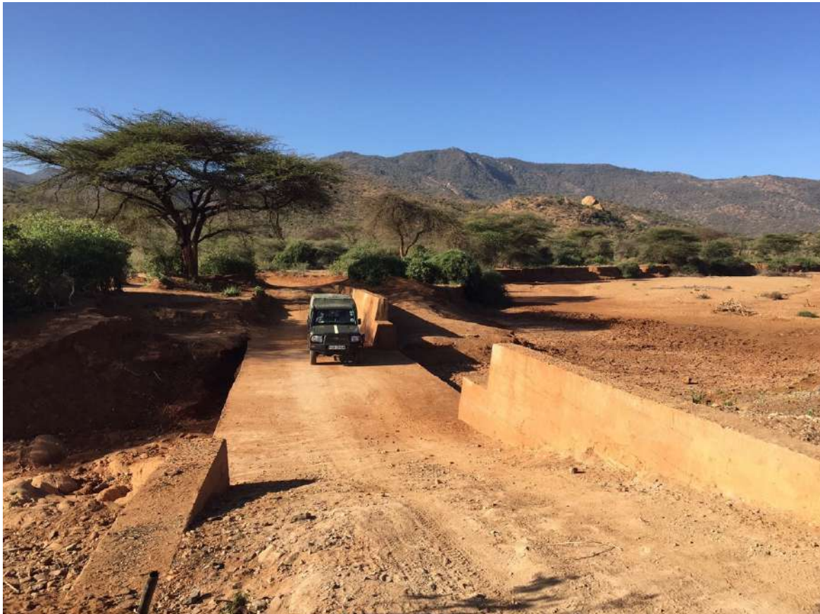
Sand dam road crossing in Lekurruki Conservancy, Laikipia, Jan 2017. [Photo Credit: David R Jordan.]
