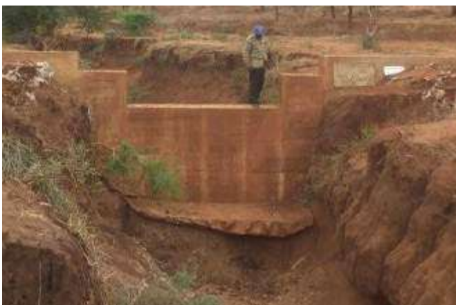
Examples of poorly constructed dam aprons
