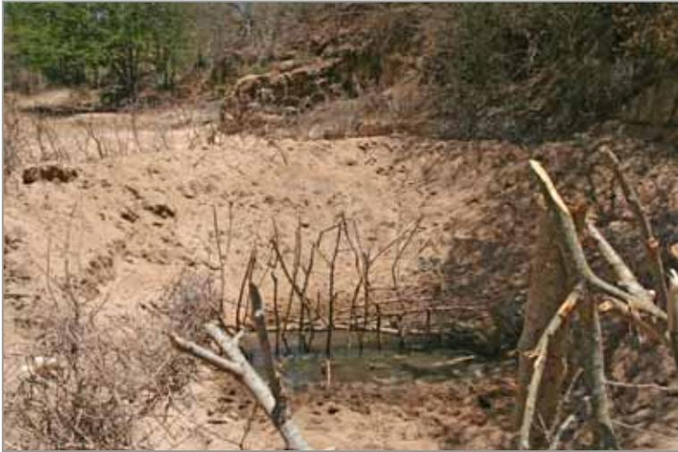
*Figure 4.1 Scoophole fenced off with thorn bush and protected against animals to reach the water*
