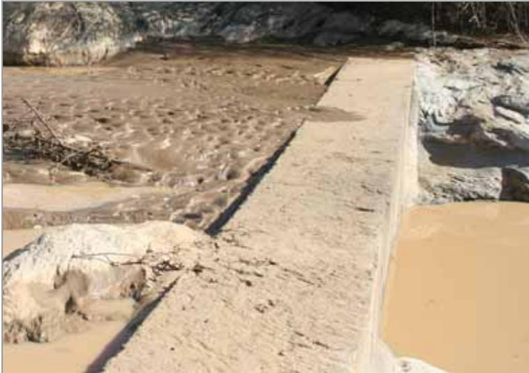
Figure 5.2 Sediment flowing over a dam
