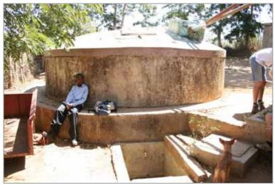
Figure 2.22 Reservoir containing rain water collected from roof
