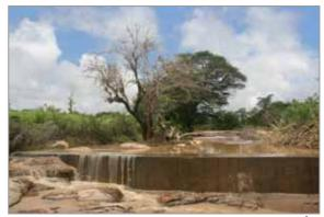
Figure 4.30 Discharge at 24 November 10:00: 0.02 m<sup>3</sup>/s
