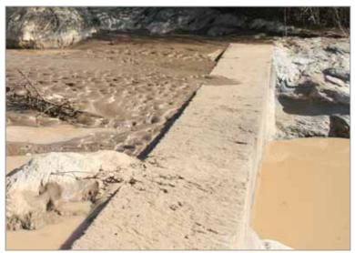
Figure 5.2 Sediment flowing over a dam
