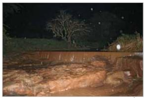
Figure 4.29 Discharge at 23 November 23:00: 0.2 m<sup>3</sup>/s
