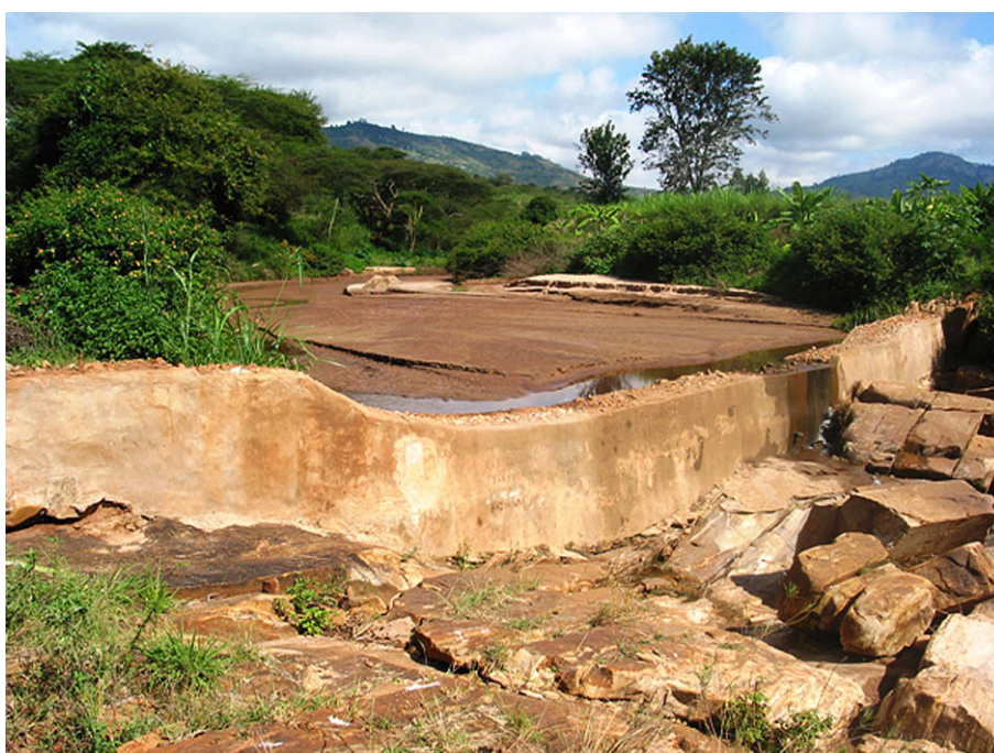
Plate 1. Typical sand-storage dam with sand reservoir upstream.
