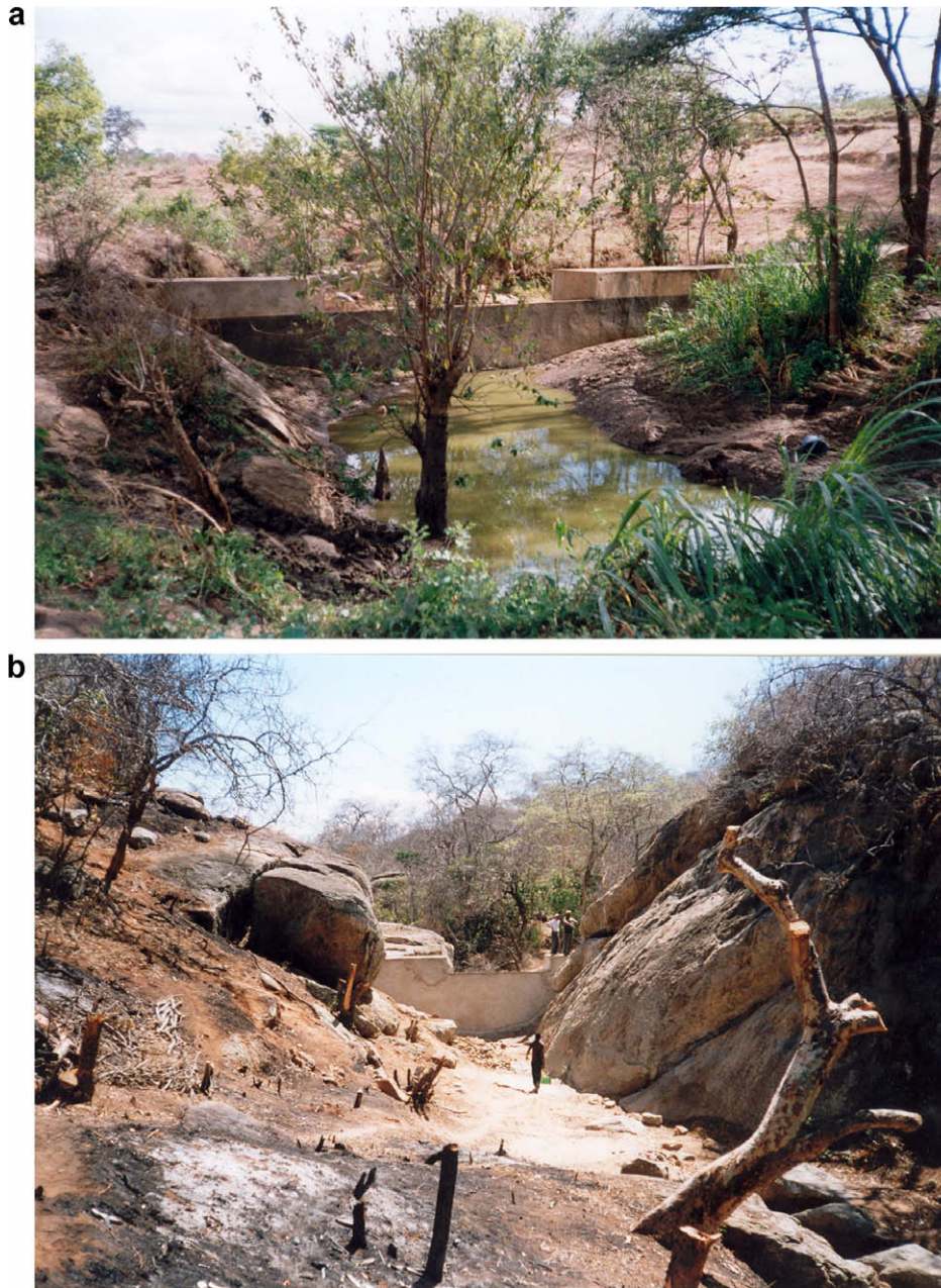
Plate 2. Two new sand-storage dams with empty upstream reservoir.
