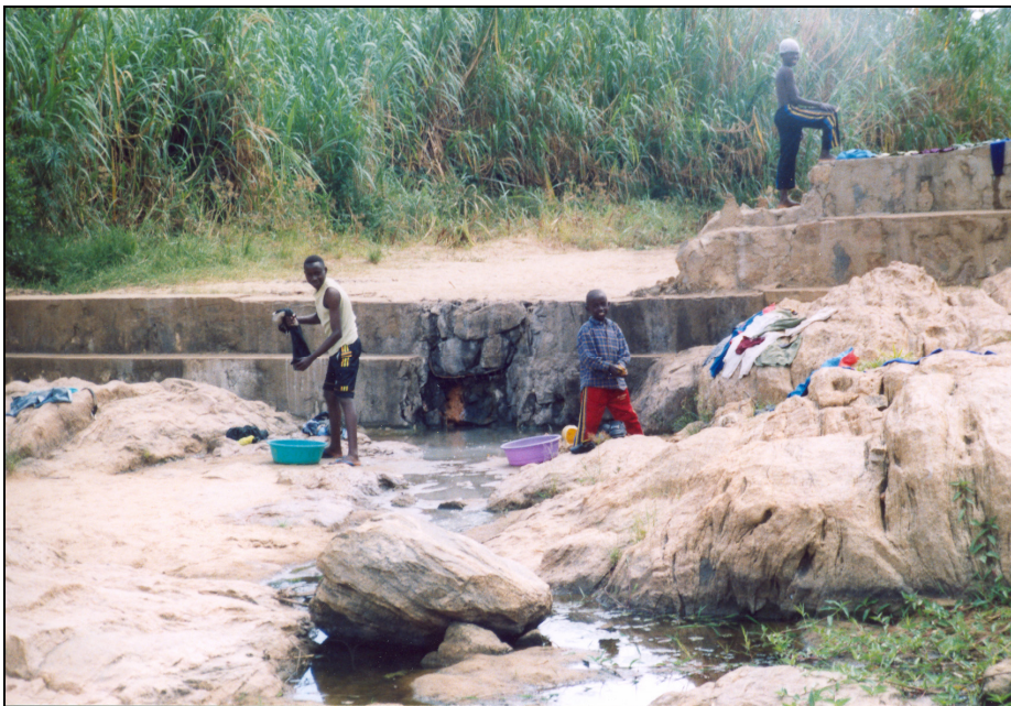
Figure 6.8: Dam with a hole in it
