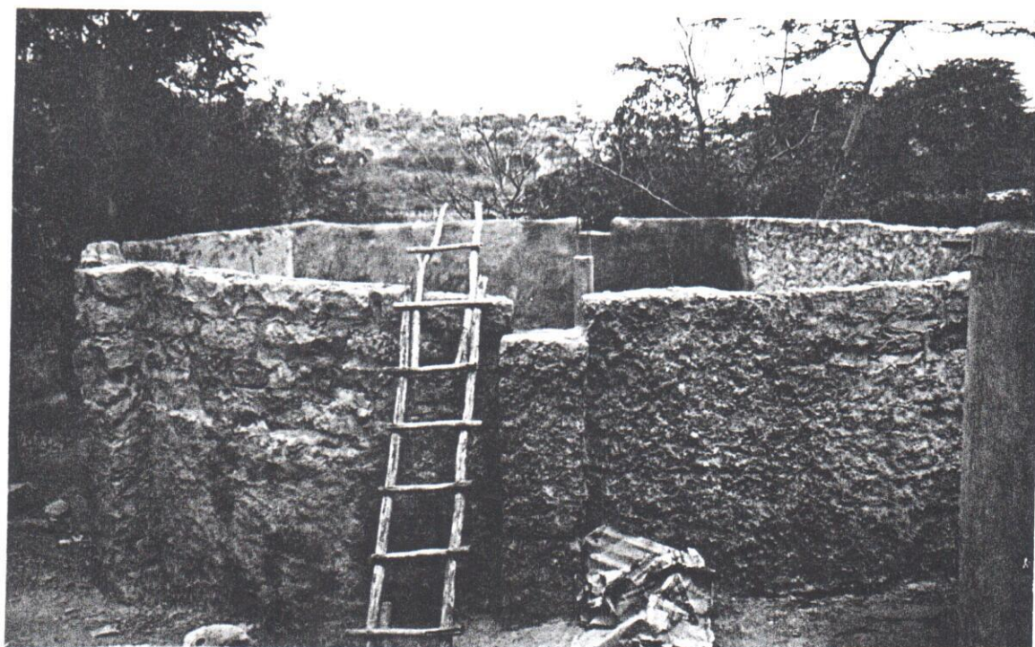
By September the Wamunyu tank had reached full height but still lacked a concrete roof and some internal plastering. The upper photo shows a trench dug for laying a pipe which will connect the tank to the borehole.
