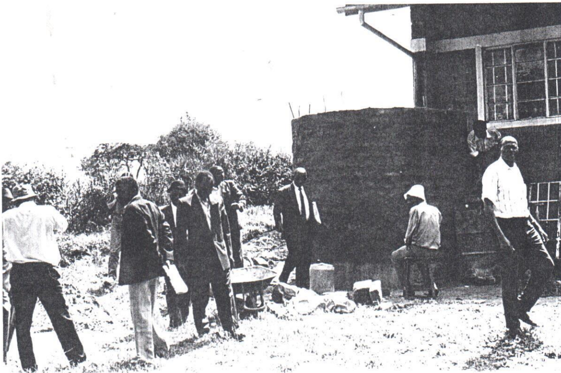
above: a small raintank under construction at Wamunyu, 13 May 97
