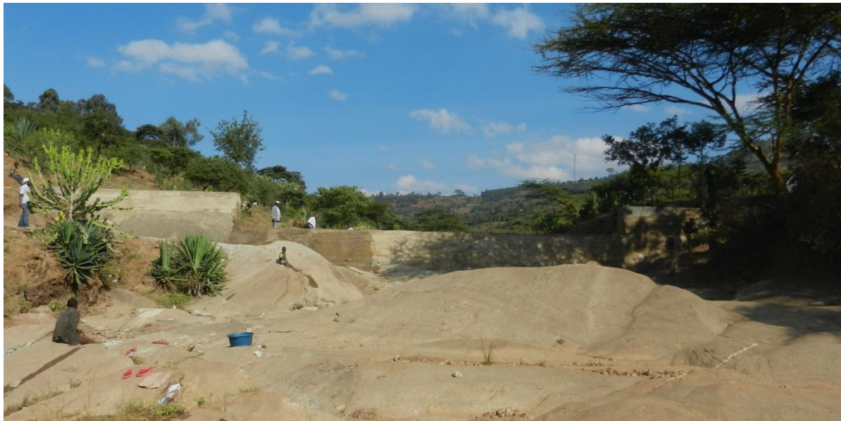
Figure 6: A newly constructed sand dam by the Kitito Self Help Group, finished in June 2013. The dam has a 17.5 meter spillway. The 1.4 meter high left wing adds an additional 7.7 meters and the right wing another 6.0 meters. It stands 2.8 meters above bedrock, is 1.8 meters thick at the base, 1.0 meter at the top of the spillway, and 0.68meters at the top of each wing. The entire structure has a volume of approximately 85 cubic meters, built by hand.
