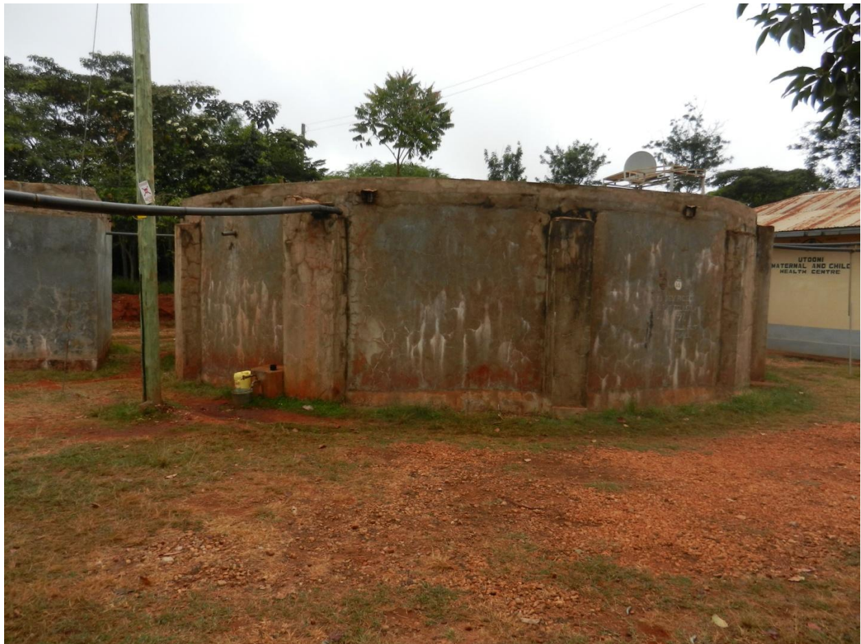
Figure 2: The UDO compound's main water storage that holds 220,000 liters. The square tank on the left holds 60,000 liters. The main office building is on the right.
