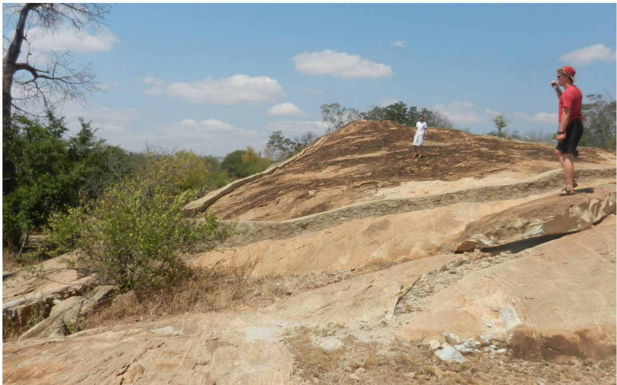
Figure 3: Catchment area of the Miamba Mitamboni SHG. The low cement and rock walls converge at a point behind the shrub in the lower left and feed into a pipe leading to the storage tanks.
