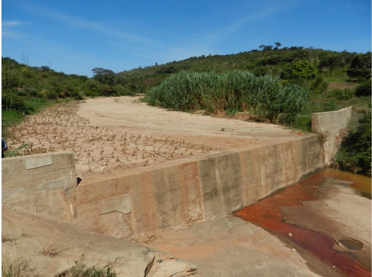
Figure 5: This sand dam was built in 2009 by the Kitandi Fruit Tree Growers SHG on the Kaiti River in Makuieni County. It was extended one year later to reach its present height. It has a 17.9 meter spillway and holds nearly 11,000 cubic meters of sand and 4,000 cubic meters of water when saturated. Note the strong stand of napier grass on the right stream bank. It is also planted as cuttings on the left bank. (Photo by the author, July 2013)
