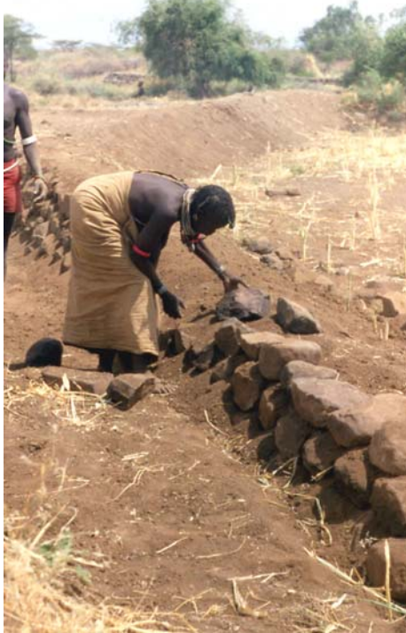
Building walls around the fields
