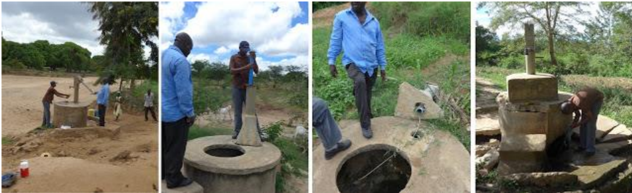
Fig. 22. Examples of pump wells. Pump well at left is functional, those to the right are broken from vandalism, floods, and general breakage.
