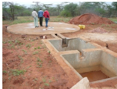
Finished surface runoffplot/ cistern
