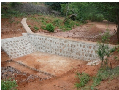
Finished sand dam
