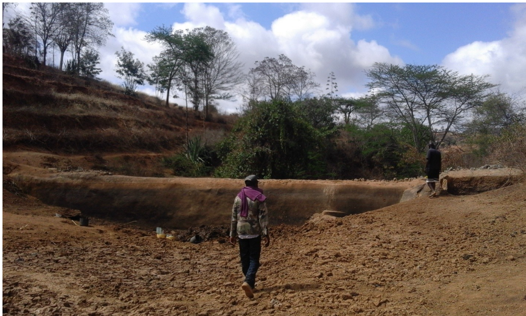
Figure 27: existing sand dam in Migwani ward, Mwingi West Sub County
