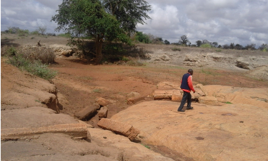
Figure 3: A sand dam located in unsuitable site that was swept away by flashfloods in Ikutha ward, Kitui South Sub County.
