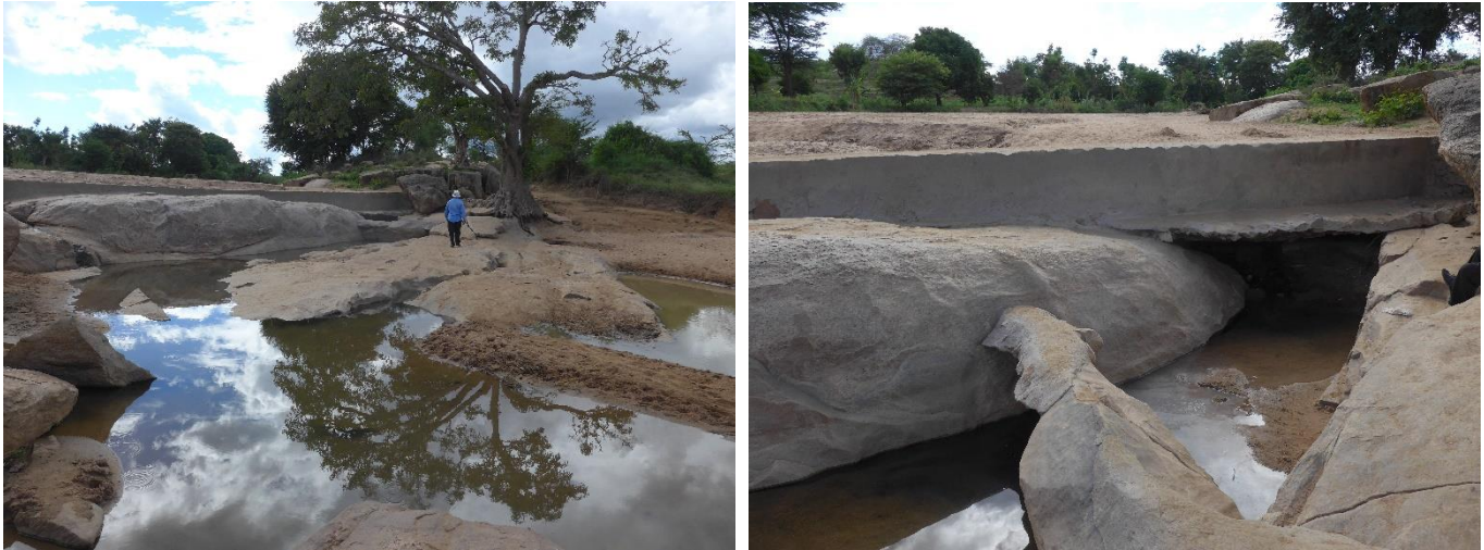
Fig. 21. Sand dam showing large degree of pooling below dam, seen actively flowing from a large hole in the dam (right panel).
