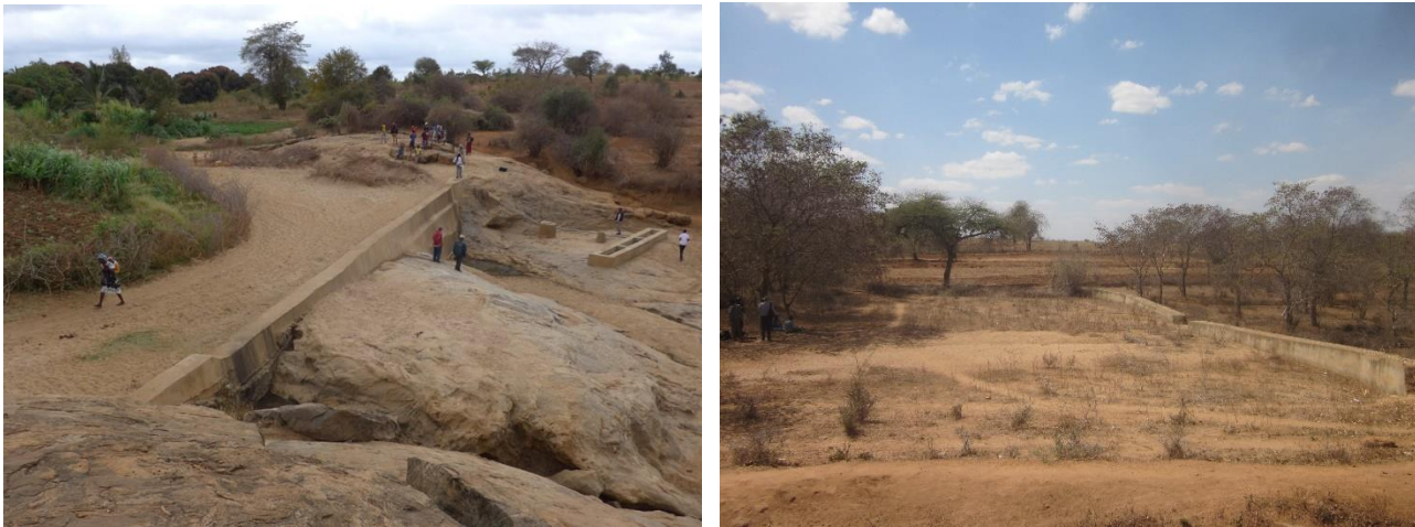
Fig. 1. Two examples of sand dams in Ukambani. Sand dam in left panel has intact dam face, functional scoop holes for water collection (in background, surrounded by brush to exclude livestock), and evidence of green vegetation. Sand dam in right panel lacks of any evidence (such as water collection site, vegetative greening) of water accumulation, and vegetation growing on sediment surfacing suggests siltation which would limit effective storage of water.
