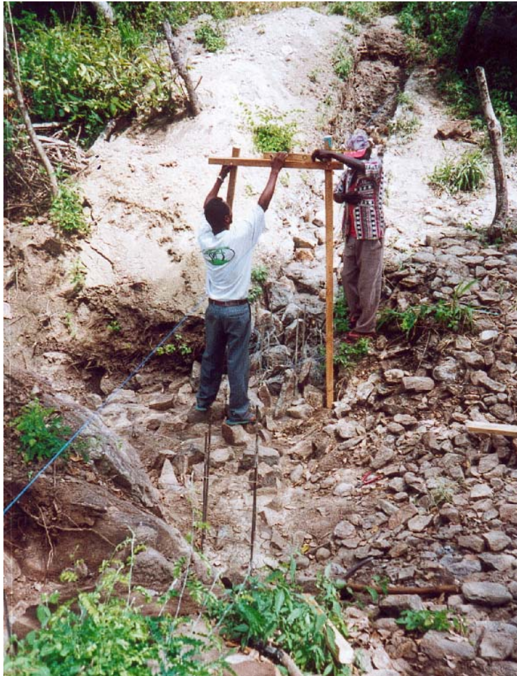
Figure 4.9: Setting wooden frames
