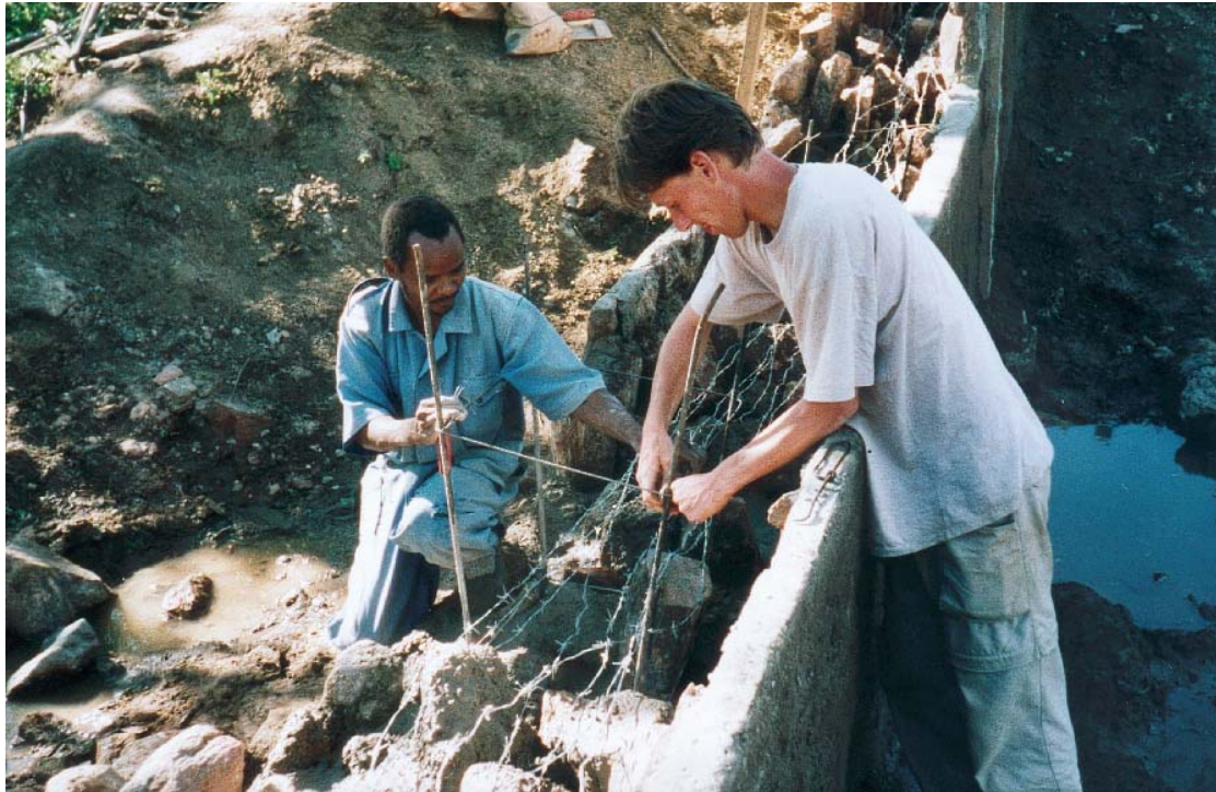
Figure 4.11: Horizontal reinforcement using barbed wire
