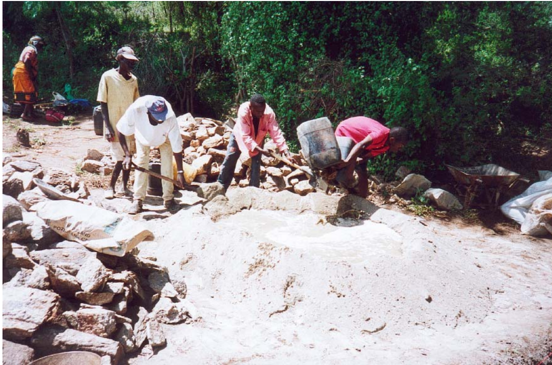
Figure 4.12: Mixing cement
