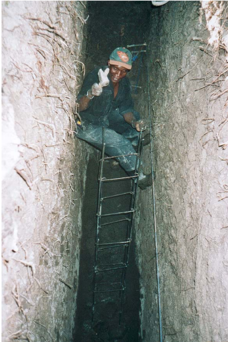
Figure 4.10: Reinforcement columns
