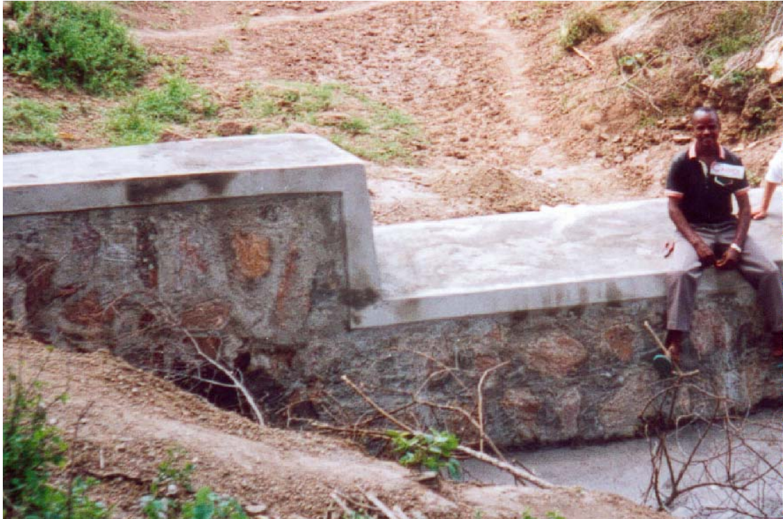
Figure 4.13: Plastering the dam is the final part of construction
