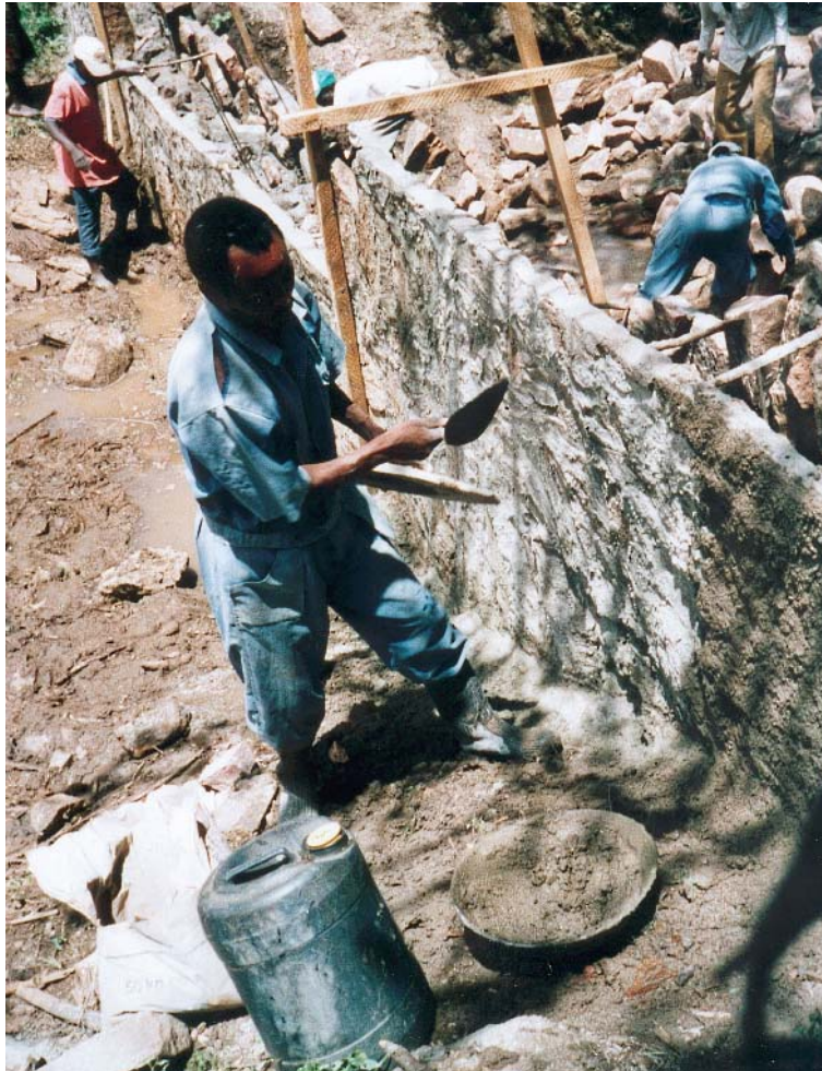
Figure 4.6: Plastering the dam
